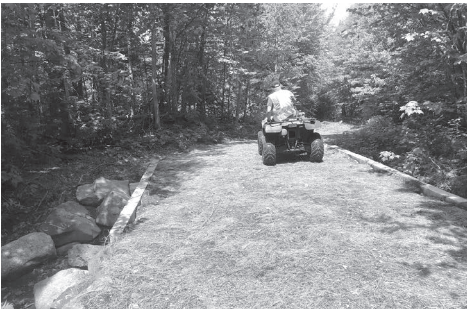
Trail Bridge Replacement Work
