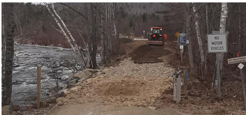
Narrow Gauge Repair- December 29, 2020, photo credit, Travis Chandler
