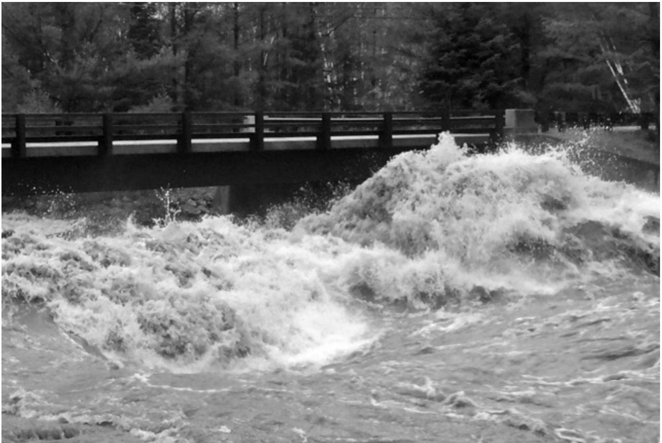
8' flood waves at Carriage Road bridge during late October flood
